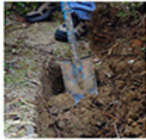
LAY OUT SYSTEM, DIG TRENCHES AND HOLES
